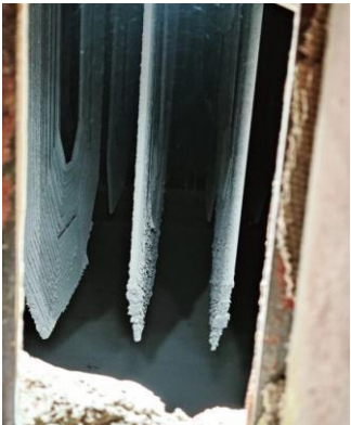
Ash Accumulation in the LTSH
