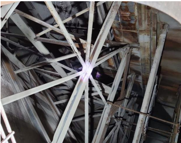
Erosion/Corrosion in APH Supports/Structural Beams at Unit A1
