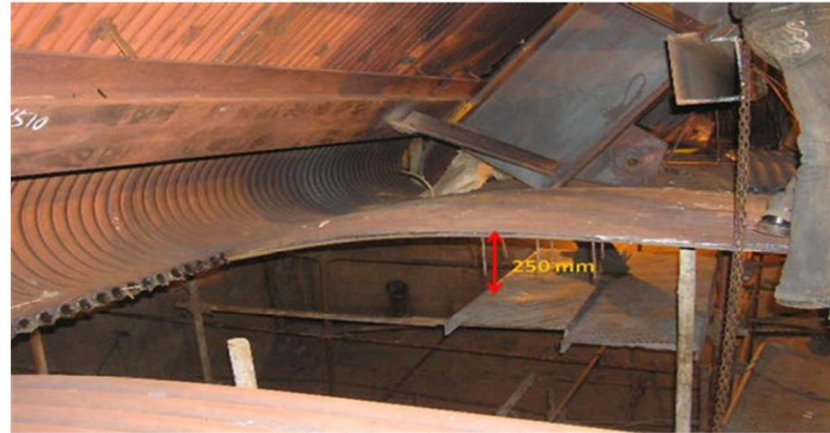
Damages to the "S" panel.
